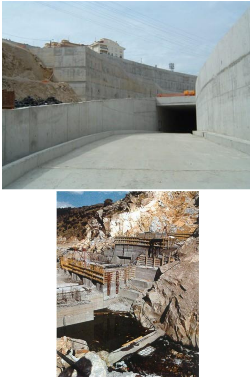
Fig. 4: Dargão Stadium Tunnel / Catapereiro Dam – excavations
