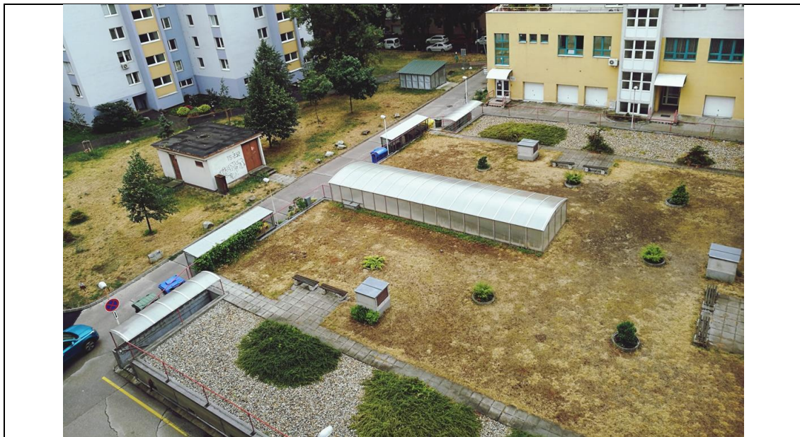
Fig. 2: Top view of the green garage roof
