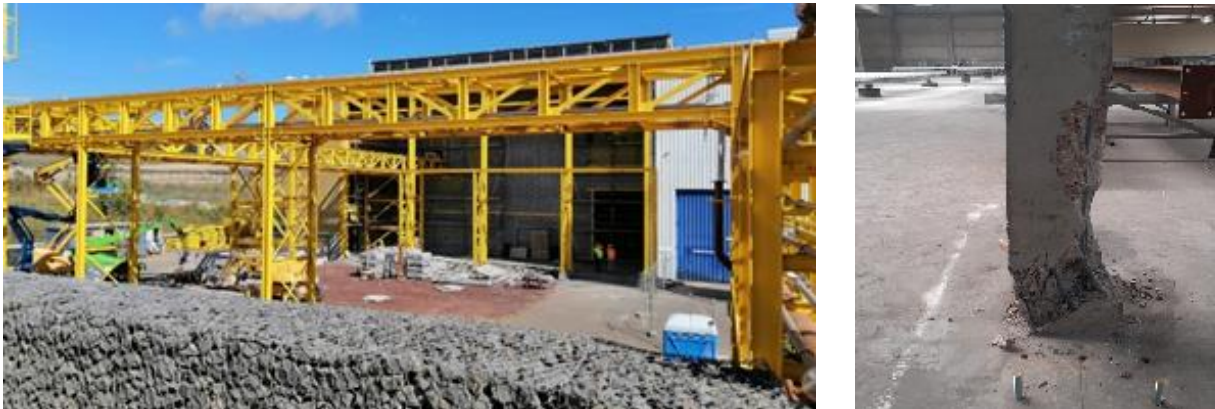
Fig. 5: Belo Jardim (Azores) Thermal Power Plant / Industrial Building (Famalicão) - structures
