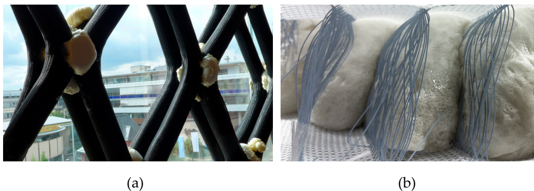
Figure 9. Textiles for free-form architectures in glass facades (reproduced from [70] under the terms and condition of CC BY-NC 4.0 license): (a) external coating composed of pressure-resistant lightweight ropes made of foamed textile sleeves, and (b) cross-sectional detail of a 3D textile-foam spacer fabric solution.
