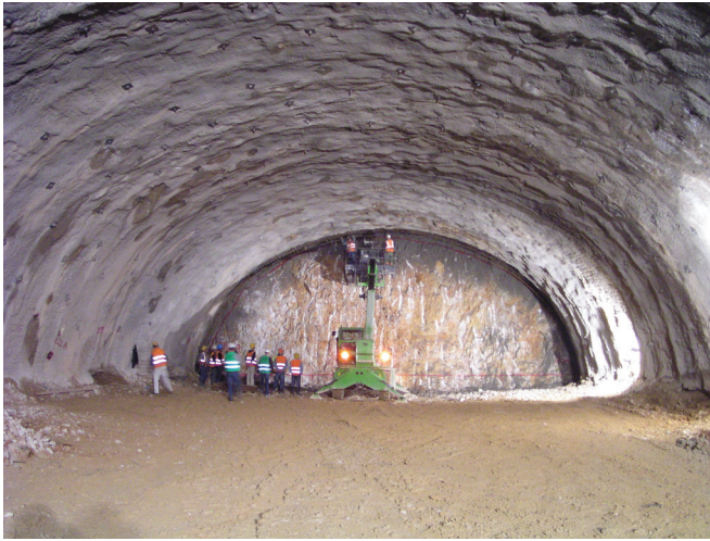
Fig. 1. Example of a tunnel construction in complex karst environment. [Colour online.]
