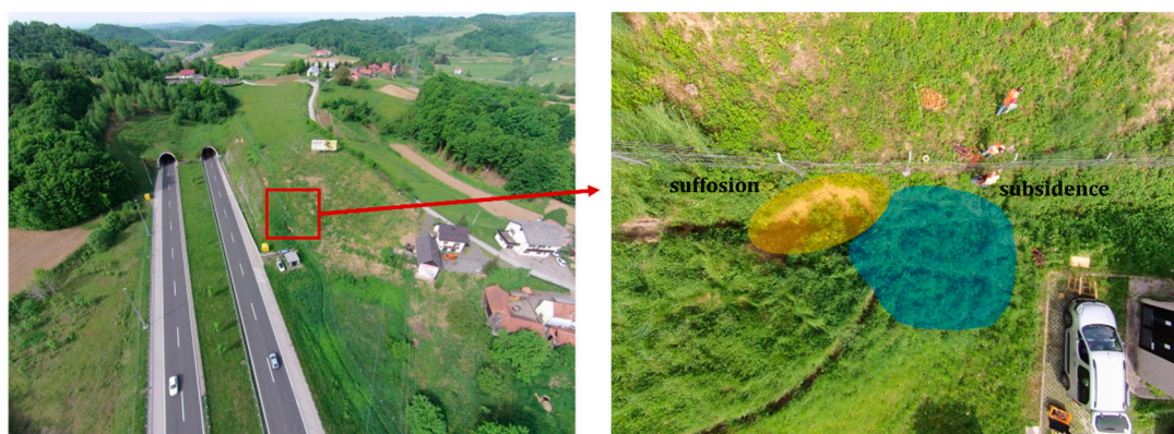
Figure 4. Suffosion next to the right side lane of Rijeka–Zagreb highway.
