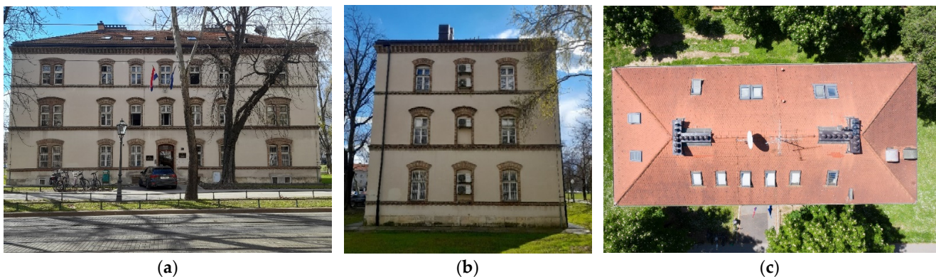
Figure 5. (a) View of the east façade; (b) View of the north façade; (c) View of the roof (photo credit: Mislav Stepinac).
