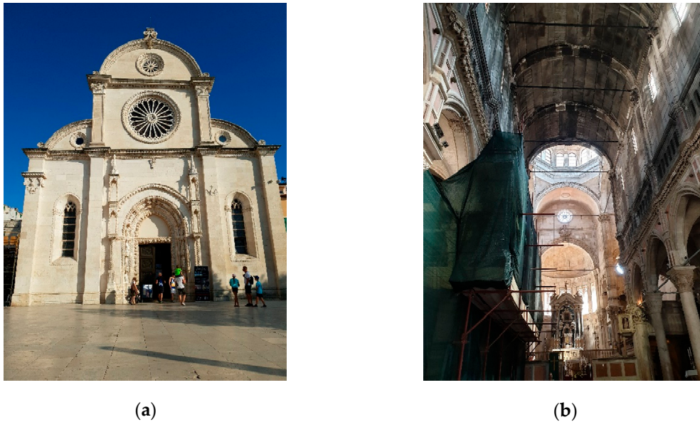
Figure 6. Cathedral of St. James in Šibenik, Croatia. (a) West view of cathedral and (b) iron tie rods inside the cathedral.
