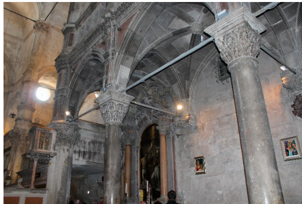
Figure 1. Cathedral of St. James in Šibenik (Croatia). Tie rods are supporting the walls and arches.
