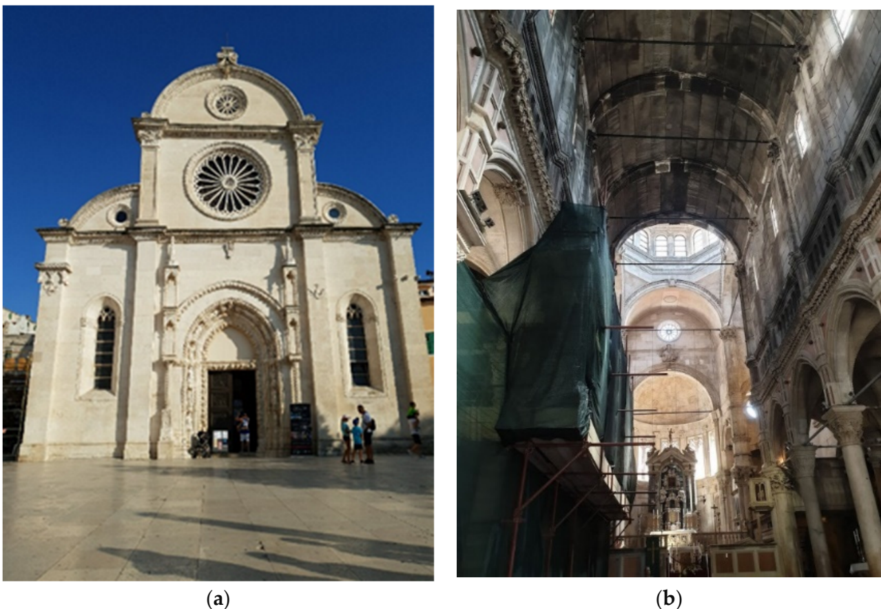
Figure 3. Cathedral of St. James in Šibenik: (a) West facade (b) System of tie rods inside.
