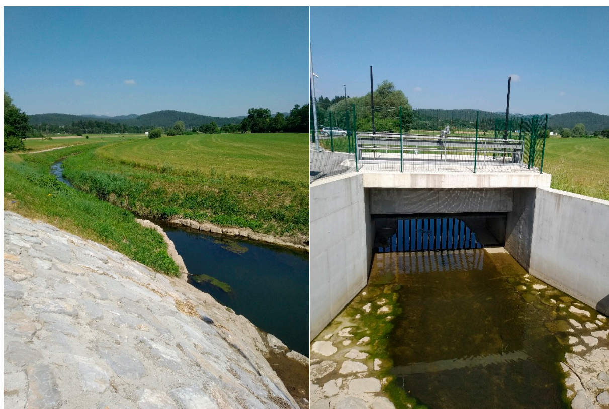
Figure 4. Left photo shows situation upstream of the hydro-technical equipment (i.e., the area that is flooded during high-flow events) and right photo shows the hydraulic structure with a gate used to retain the water during the floods. Brdnikova reservoir is shown.
