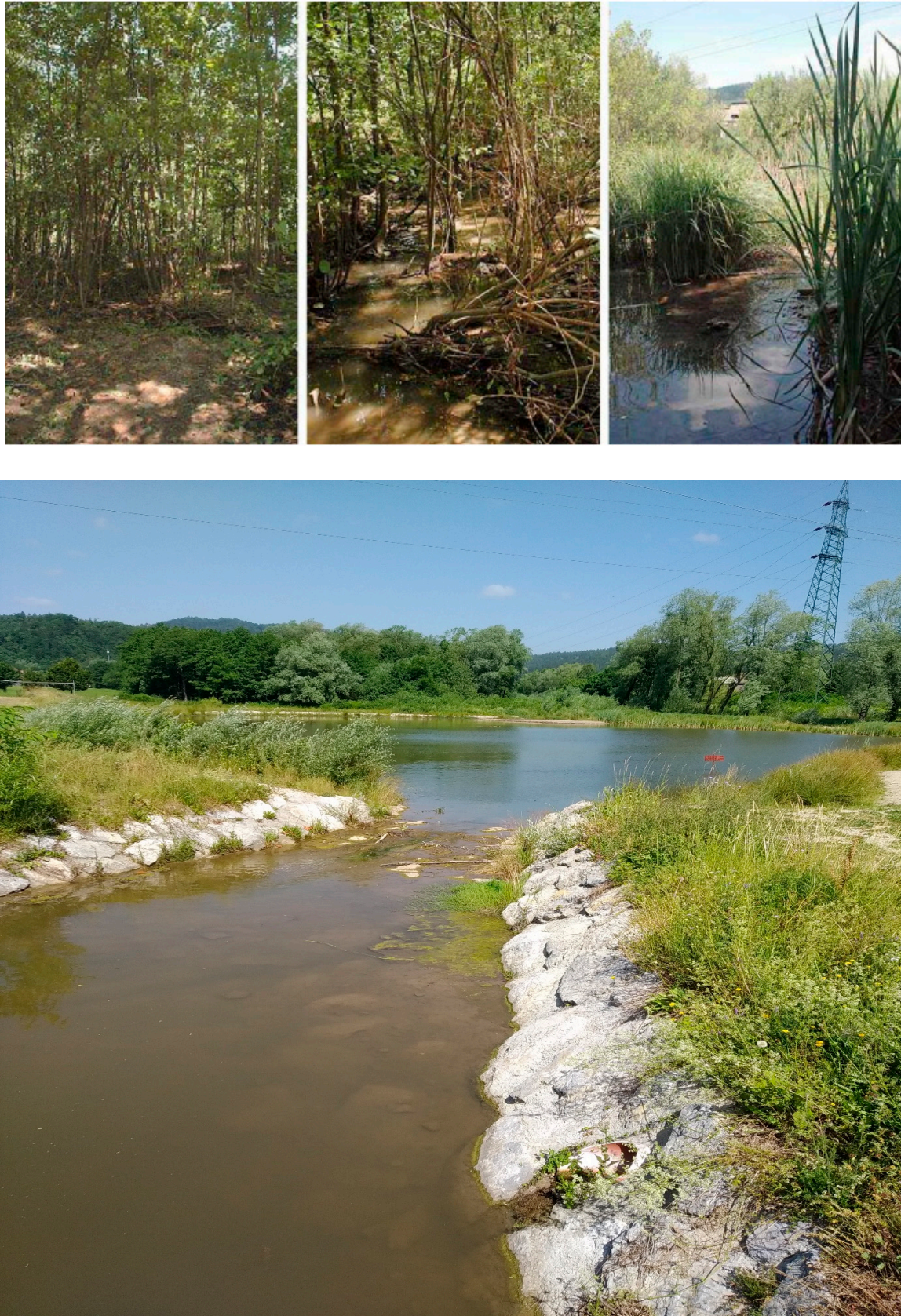
Figure 3. The upper three photos show situation in the Podutik reservoir before maintenance carried out in 2019 (adopted after Replik [46]) and lower photo shows situation in year 2021.
