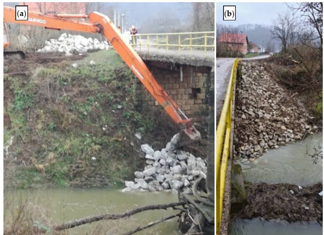
Figure 15. Immediate measures to secure the abutment of Matija Gubec street bridge: (a) beginning of the work; (b) completed infill.
