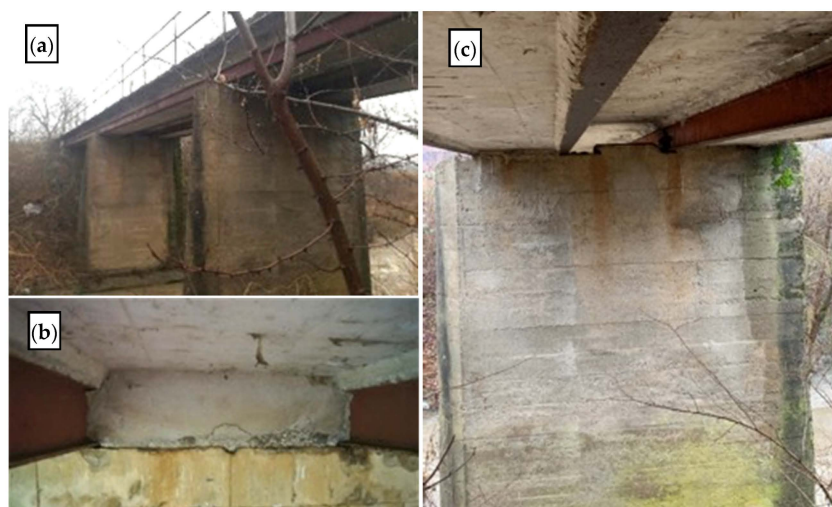
Figure 12. Nikola Tesla street bridge: (a) view of the bridge; (b) main girders to abutment support; (c) superstructure under view.
