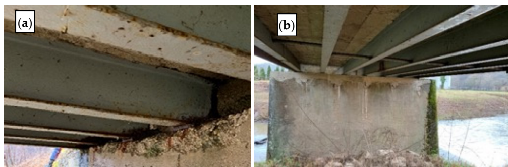
Figure 11. Svračica bridge main girder support: (a) abutment; (b) column.
