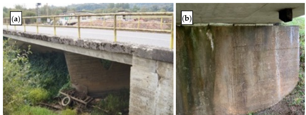
Figure 10. Maja bridge: (a) side view of the bridge; (b) abutment wall.
