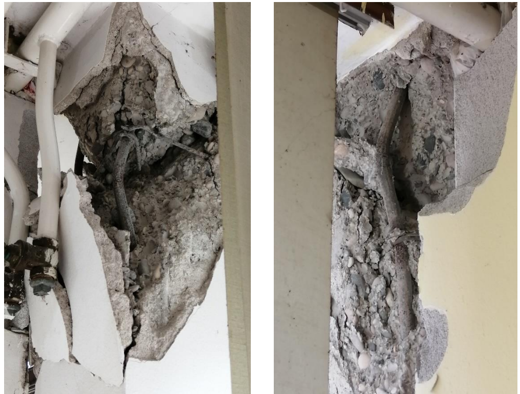
Figure 1. Buckling of plain bar reinforcement on top of the RC piers.
