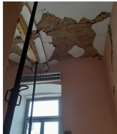
Vault damage/collapse
