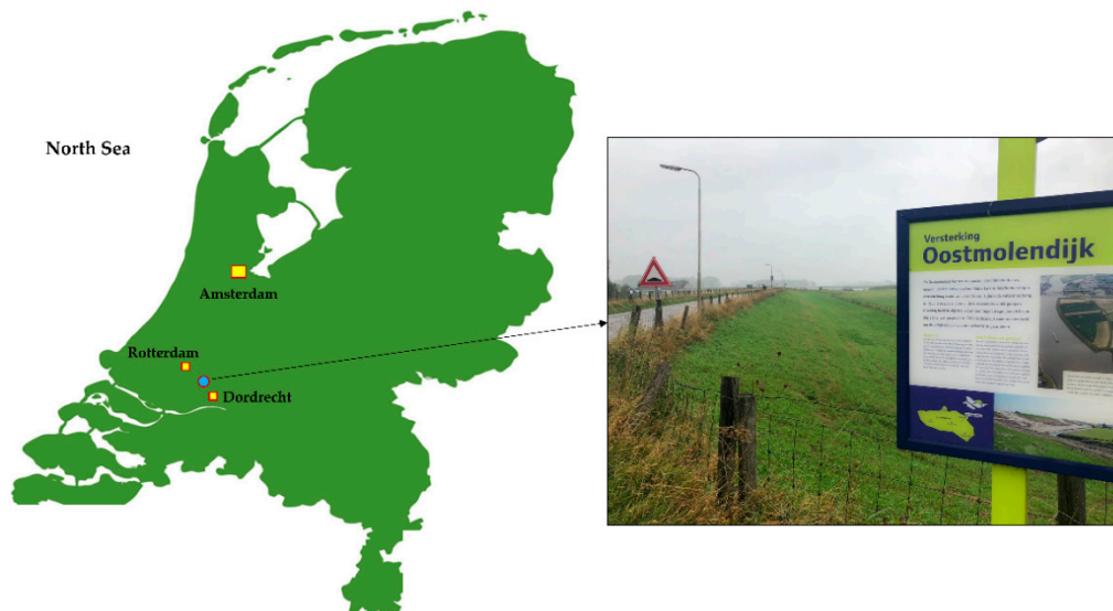
Figure 7. Location of the case study embankment Oostmolendijk.
