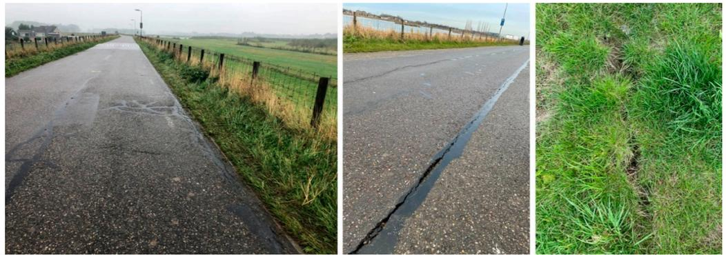
**Figure 8.** Presence of cracks on the embankment road and slopes.
