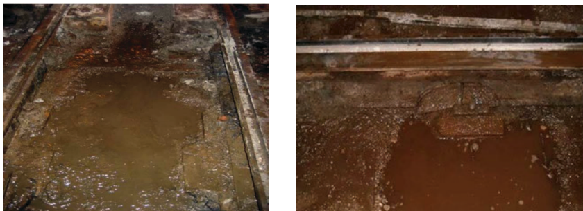
Figure 3. Condition of the closed track formation during the most part of year
