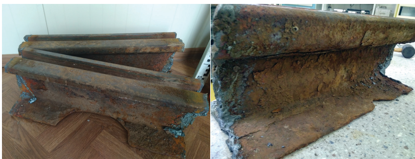
Figure 2. Rail degradation noticed at urban tracks
