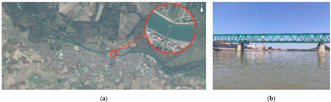
Figure 1. Orthophoto map of the case study area (a), photo of the bridge (b).
