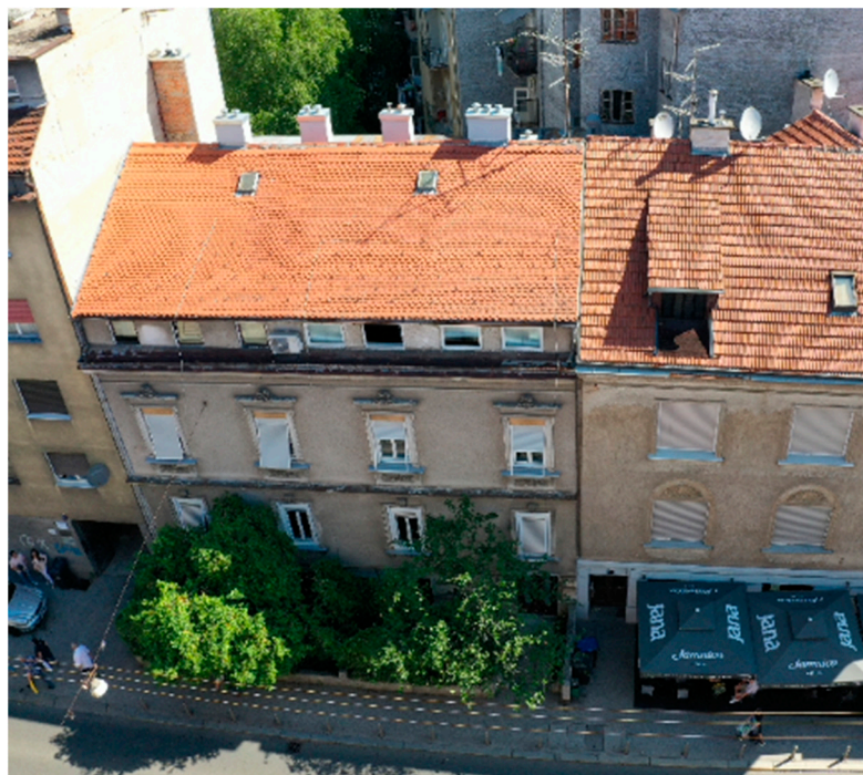
Figure 6. Residential building in Zagreb.
