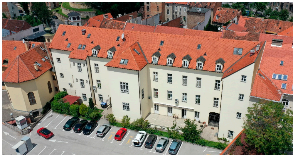
Figure 7. Educational building in Zagreb.
