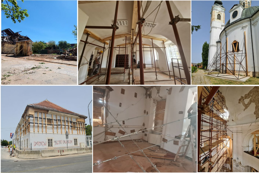
Fig. 15 Demolition and emergency measures in heritage buildings
