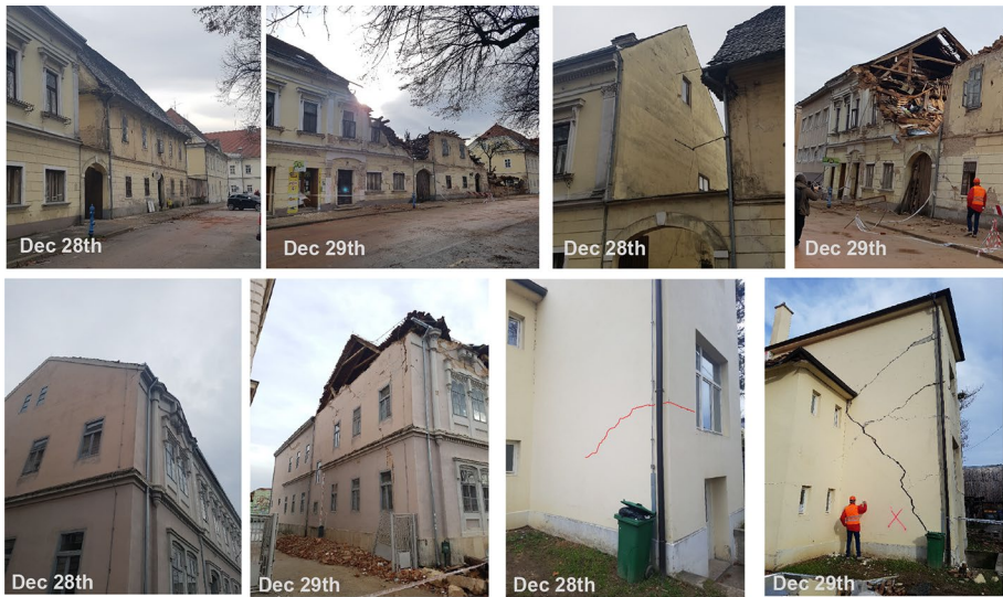
Fig. 27 Comparison of damage to buildings in Petrinja following the foreshock (indicated with Dec 28th) and the main shock (indicated with Dec 29th)
