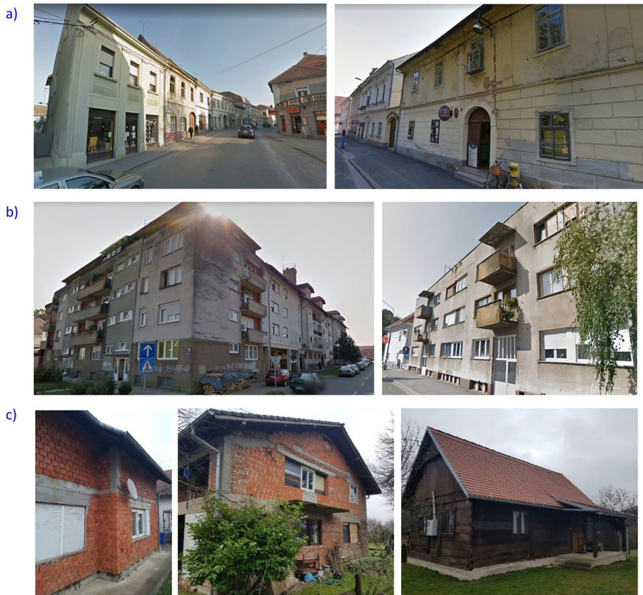
Fig. 2 City of Petrinja a URM buildings in the historic centre, b Multi-apartment masonry buildings, and c Single masonry and wooden residential buildings (Google Maps 2021, CCEE 2022)
