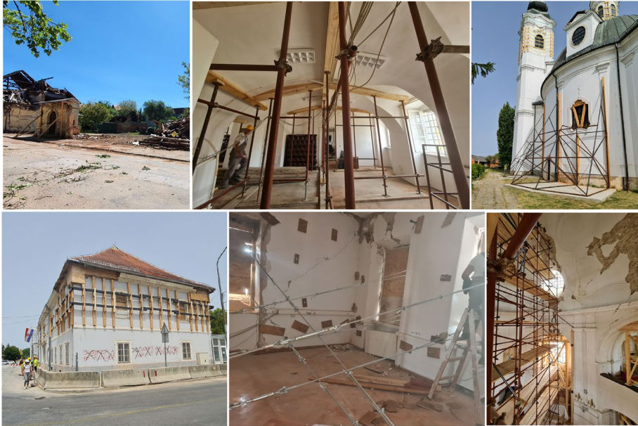
Fig. 15 Demolition and emergency measures in heritage buildings
