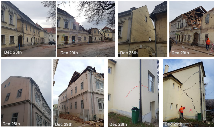
Fig. 27 Comparison of damage to buildings in Petrinja following the foreshock (indicated with Dec 28th) and the main shock (indicated with Dec 29th)
