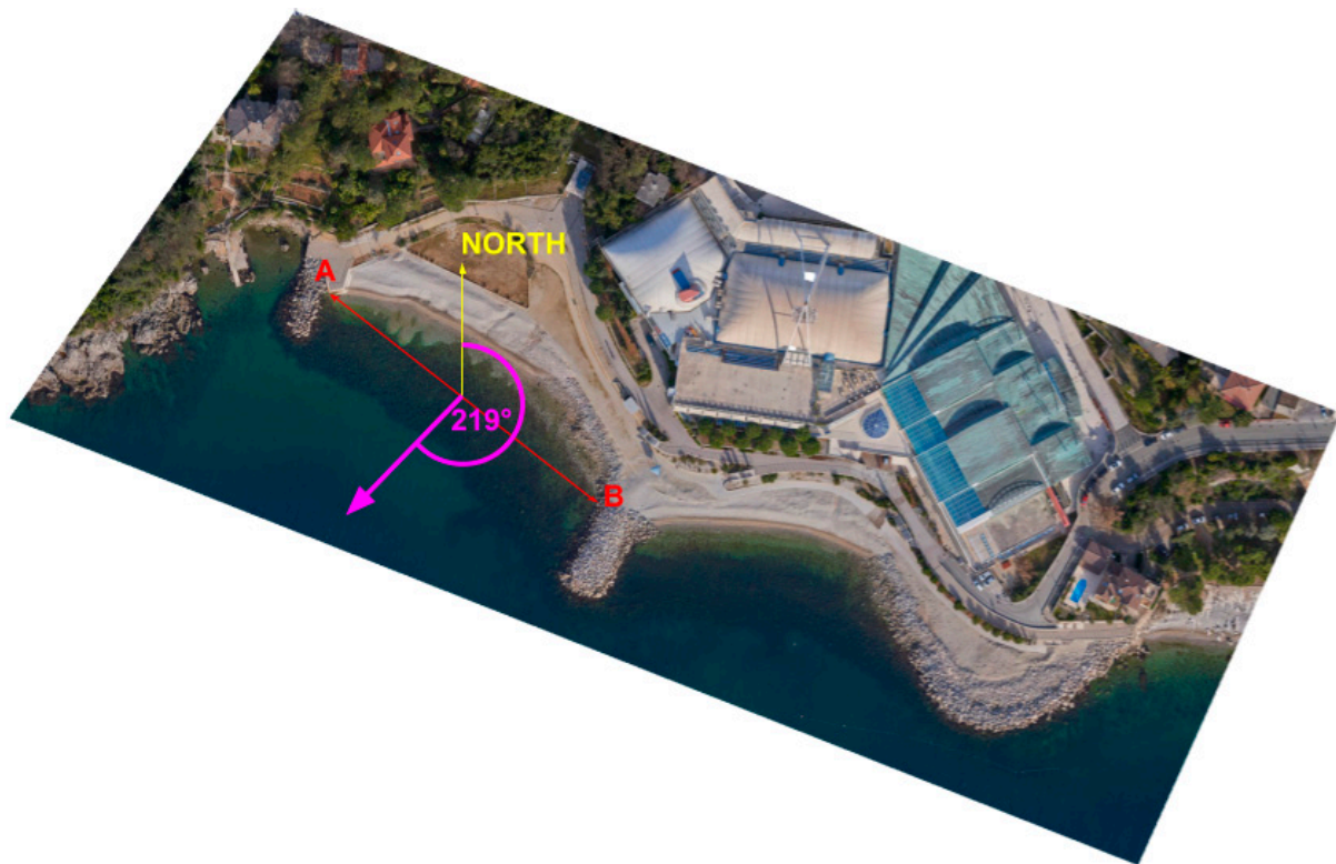
Figure A3. Aerial picture of Ploče beach showing a red line connecting end points (A and B) of the western beach cell, a yellow arrow pointing north, and a purple arrow perpendicular to the red line connecting beach endpoints (A and B) and in the direction of the beach orientation, which closes an angle of 219^\circ from north.
