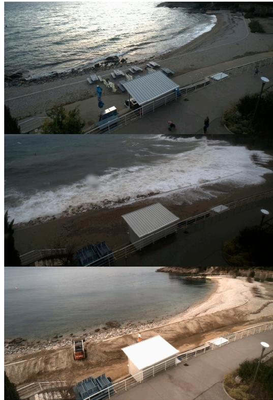
**Figure 11.** Images from the video-monitoring system depicting wave conditions during the G13\_G14\_K1 event (**top**), G17\_G18\_K3 event (**middle**) with visible overtopping on Profile 1, and workers removing the overwashed sediment on 9 January 2021 (**bottom**)—5 days before the 18th geodetic survey took place, and 2 weeks after wave event G17\_G18\_K3.
