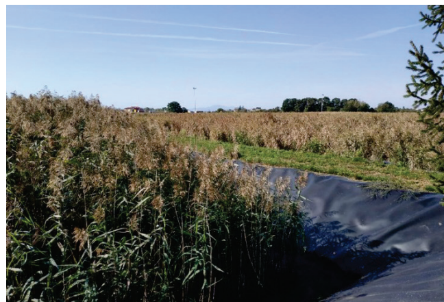
Figure 4 Constructed reed beds within WWTP Cakovec
