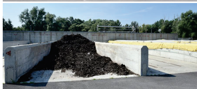
Figure 5 Constructed composting plant within WWTP Varazdin
