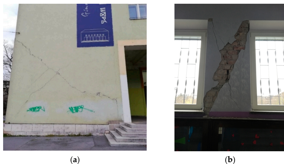
Figure 3. Observed characteristic damages on (a) the load bearing walls (b) the walls between the openings.
