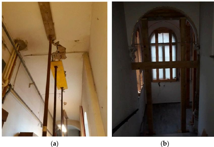
**Figure 4.** Emergency interventions taken to ensure the stability of (a) damaged vaults and (b) staircases.
