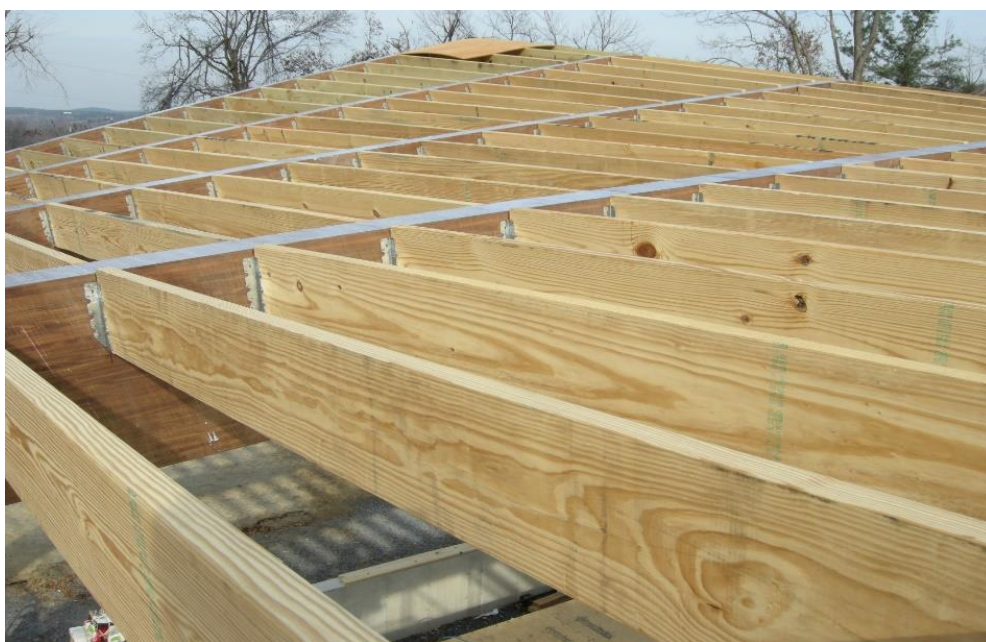
Slika 1.1 Prikaz linijskog nosača (Izvor: [ http://unalam.blogspot.com/2015/10/joist-wednesdays-word-of-week.html?q=girders ])
