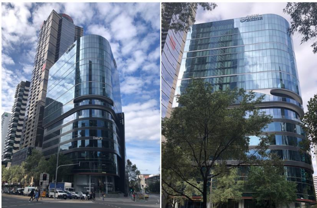
Slika 1.7. Southbank building – Melbourne, Australija
